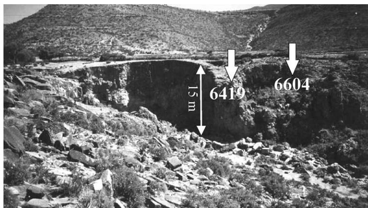
Fig. 5. Location of soil samples, indicated by sample number, on Tsigaba dam. The dam is approximately 15 m high.
